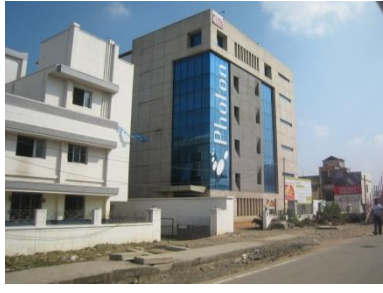
IT Corridor, Chennai
