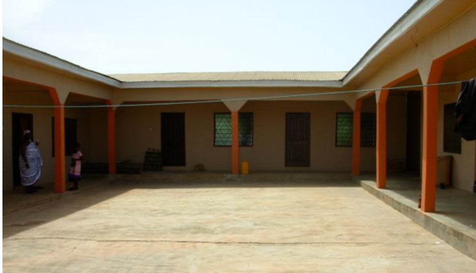
Figure 16 Interior of newly built palace for the Mantia Stool that draws on the traditional form of an open courtyard surrounded by open and closed front rooms. (Image credit: Catherine Hale)
