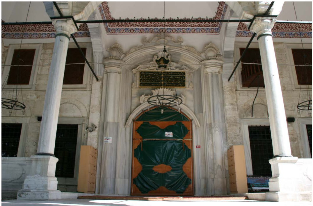
Figure 460. Selimiye Mosque, main entrance.
