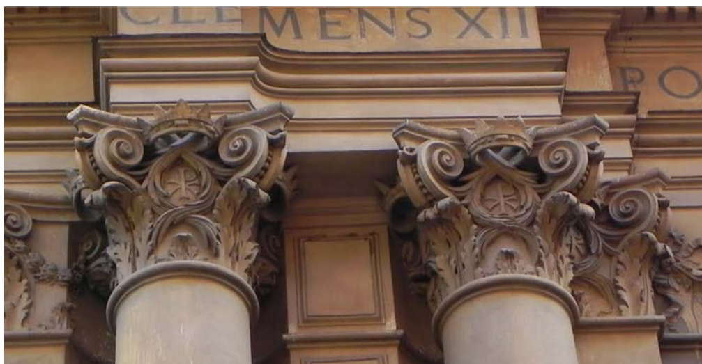
Figure 98. Column capitals of Santi Celso e Giuliano. © http://spenceralley.blogspot.com .
