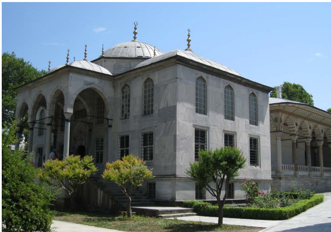
Figure 22. Library of Ahmed III, Topkapı Palace, Istanbul, 1719.
