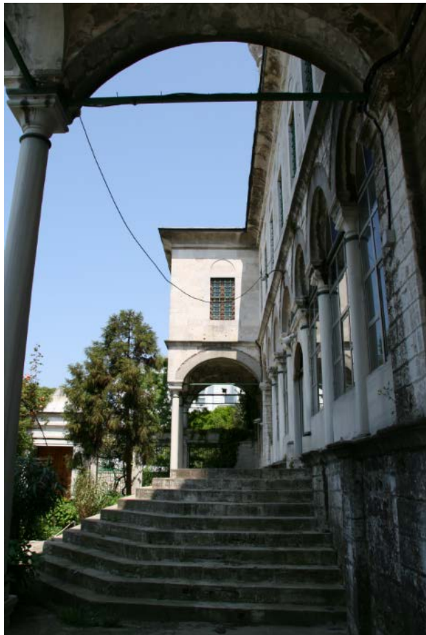
Figure 401. Beylerbeyi Mosque, lateral view of the front of the sultan's pavilion.
