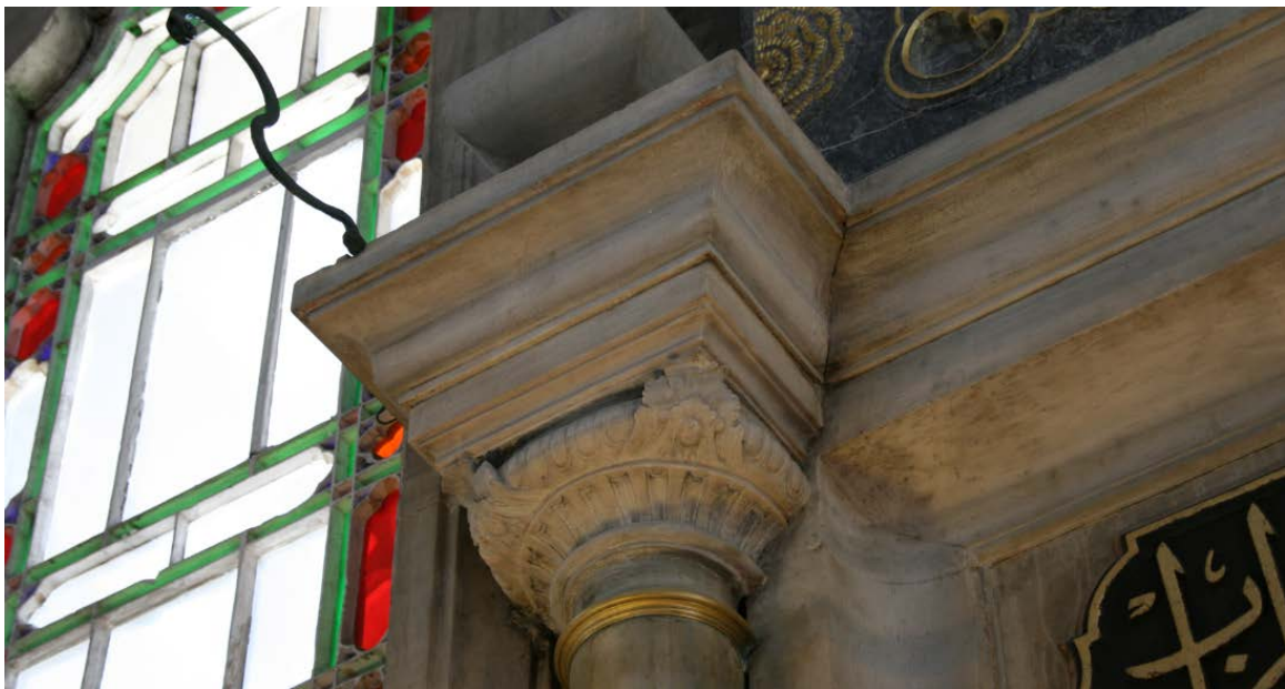
Figure 305. Laleli Mosque, column capital of the mihrab.
