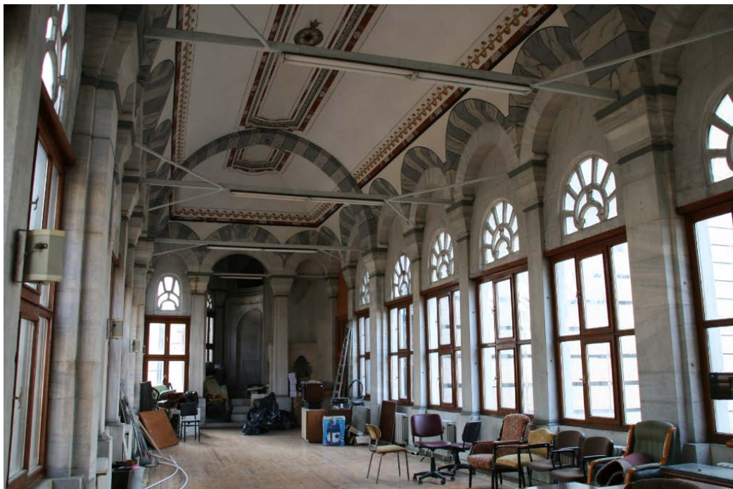
Figure 162. Nuruosmaniye Complex, sultan's pavilion, interior of the elevated gallery looking towards the entrance to the royal loge.
