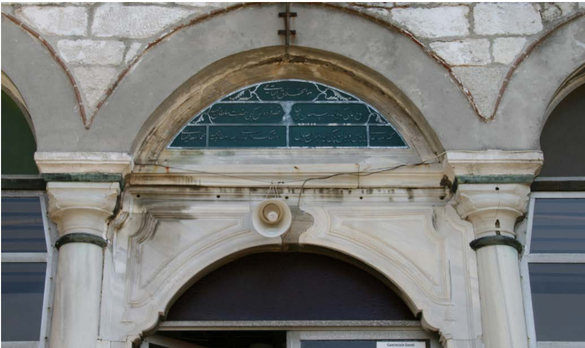
Figure 405. Beylerbeyi Mosque, inscription over the main entrance.
