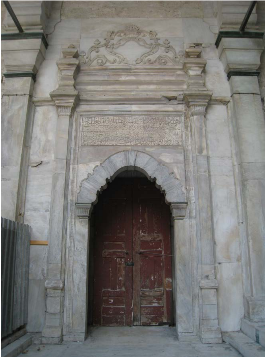
Figure 189. Nuruosmaniye Mosque, courtyard interior, lateral door.
