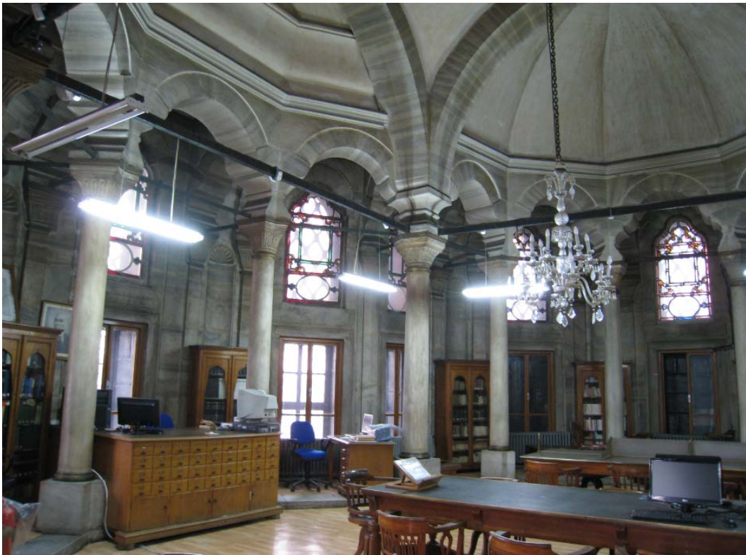
Figure 129. Nuruosmaniye Complex, library interior.
