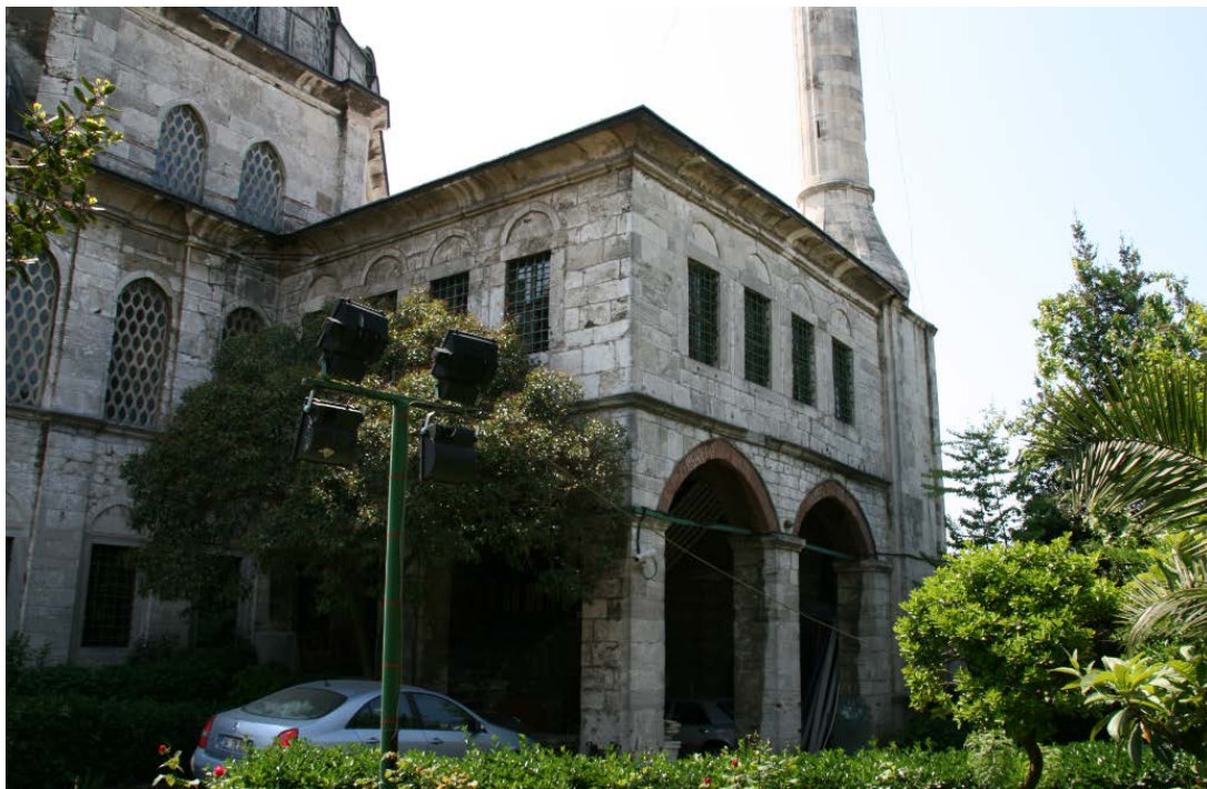
Figure 399. Beylerbeyi Mosque, looking towards the entrance block of the sultan's pavilion.
