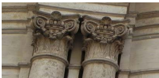
Figure 99. Column capitals of Oratorio SS. Sacramento (architect: Domenico Gregorini), Rome, 1727–30. © http://spenceralley.blogspot.com .
