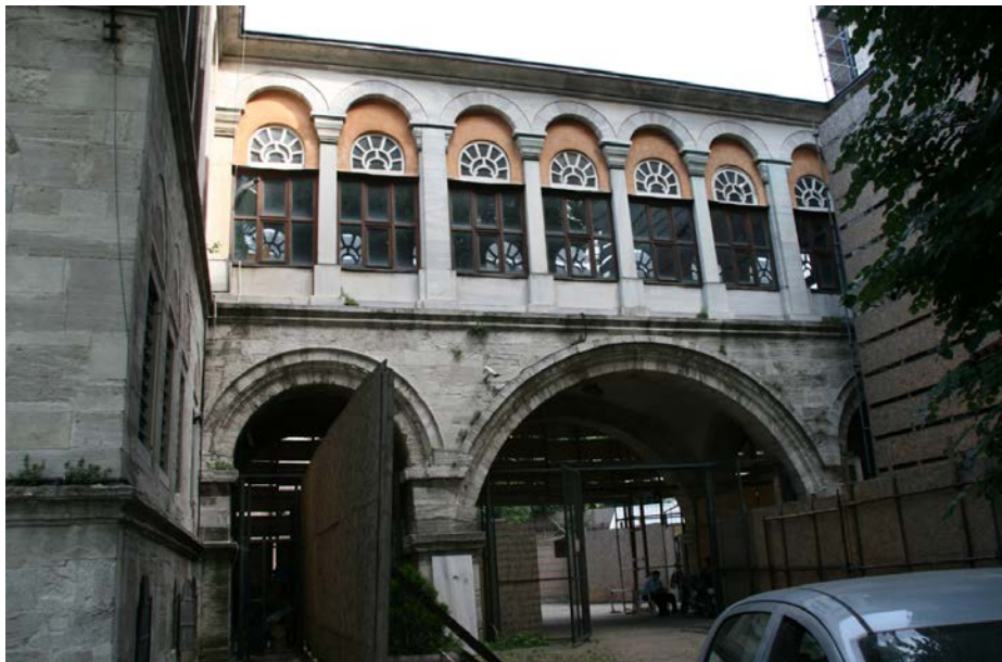
Figure 156. Nuruosmaniye Complex, sultan's pavilion, elevated gallery viewed from the back.
