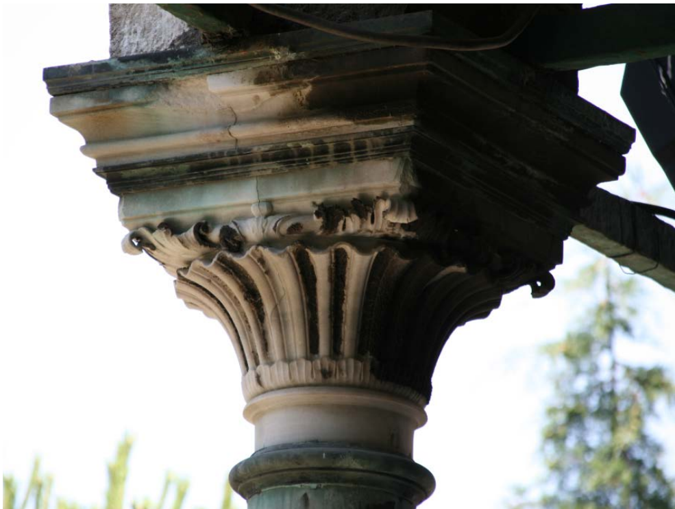
Figure 241. Ayazma Mosque, column capital of the entrance portico.
