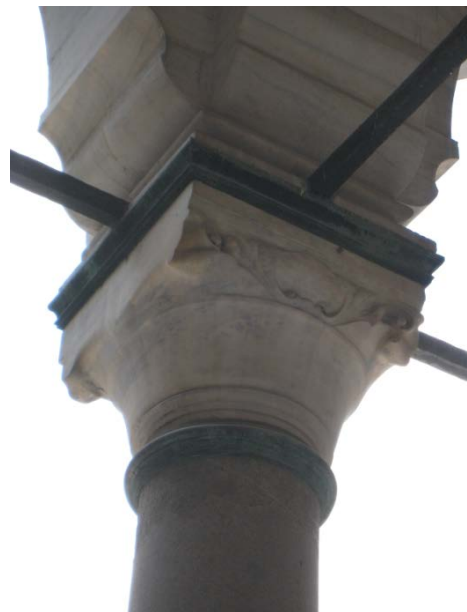
Figure 203. Nuruosmaniye Complex, unfinished column capital inside the courtyard.
