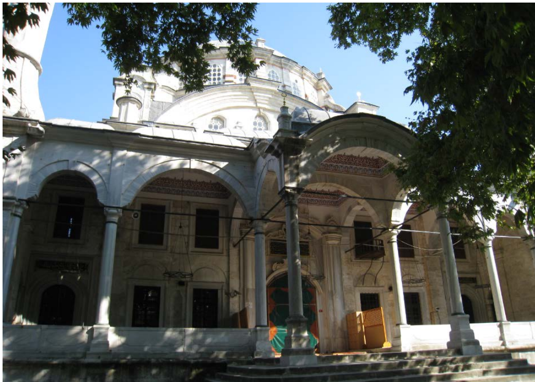
Figure 458. Selimiye Mosque, entrance portico.
