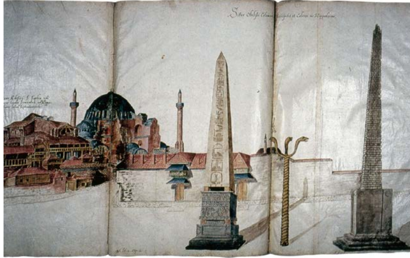
Figure 17. View of the hippodrome showing the Serpent Column before the removal of its heads. From the Freshfield Album, c. 1754. Trinity College, University of Cambridge, MS.O.17.2, fol. 20.
