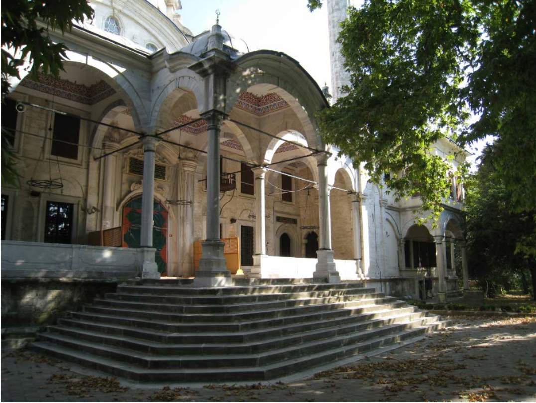
Figure 459. Selimiye Mosque, entrance portico and stairway.
