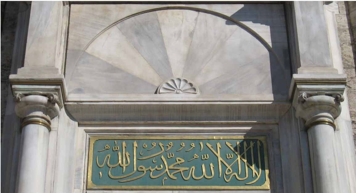
Figure 290. Laleli Mosque, courtyard exterior, pediment of the main entrance.
