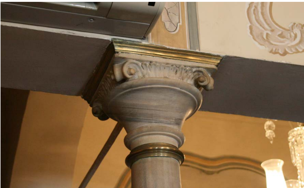
Figure 381. Hamidiye Complex, column capital inside the library.
