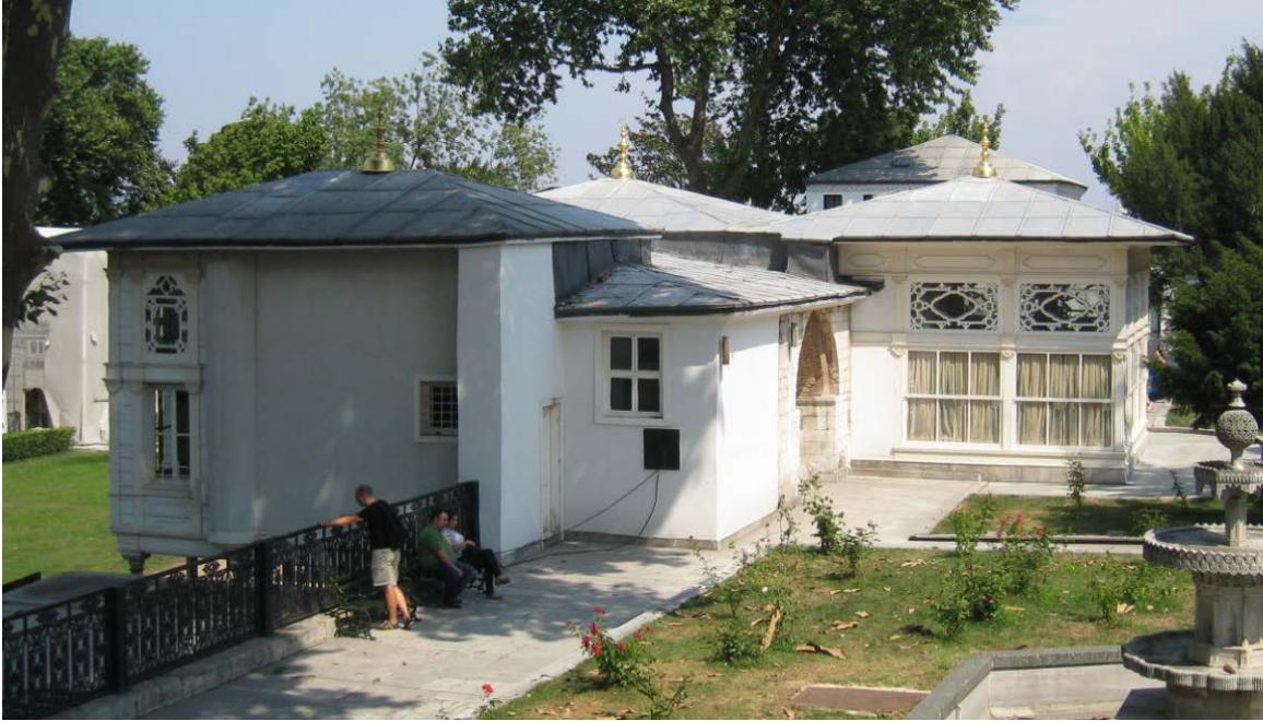
Figure 110. Sofa Kiosk, Topkapı Palace, Istanbul, built 17th century, remodeled 1752.
