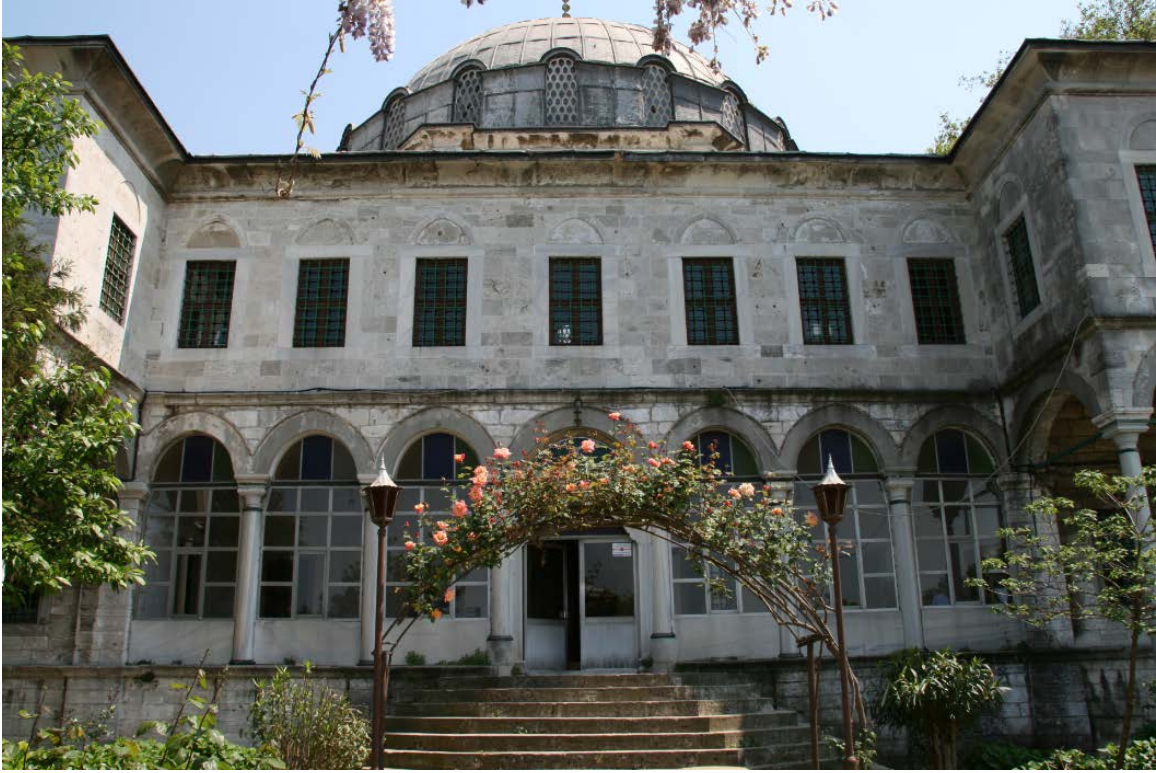
Figure 404. Beylerbeyi Mosque, pavilion façade.
