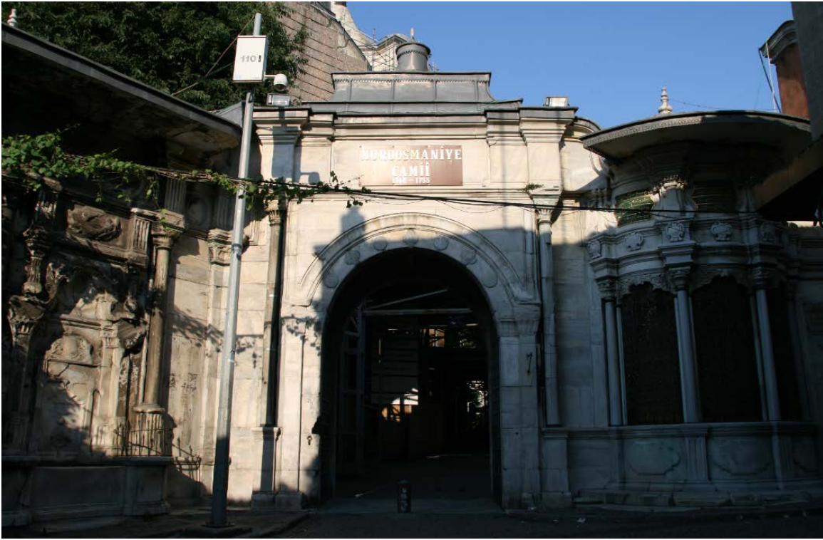
Figure 124. Nuruosmaniye Complex, west (Grand Bazaar) gate, flanked by the fountain and sebil.
