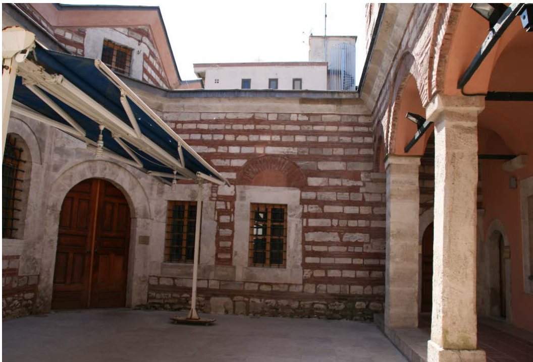
Figure 276. Laleli Complex, imaret, courtyard interior.
