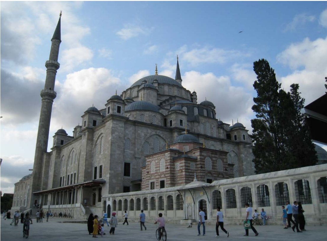
Figure 337. Fatih Mosque, with the Library of Mahmud I and one of the wall fountains of Nişancı Ahmed Pasha in front.
