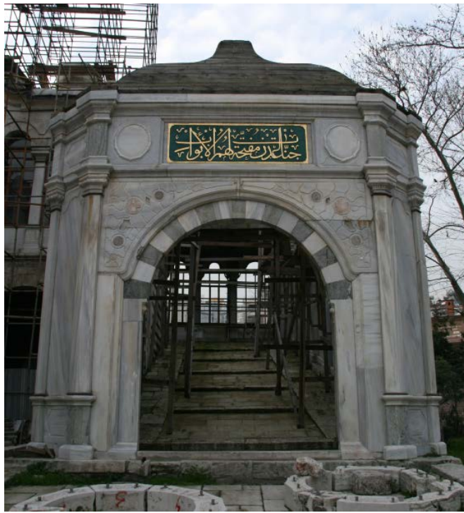
Figure 284. Laleli Mosque, entrance to the sultan's pavilion.
