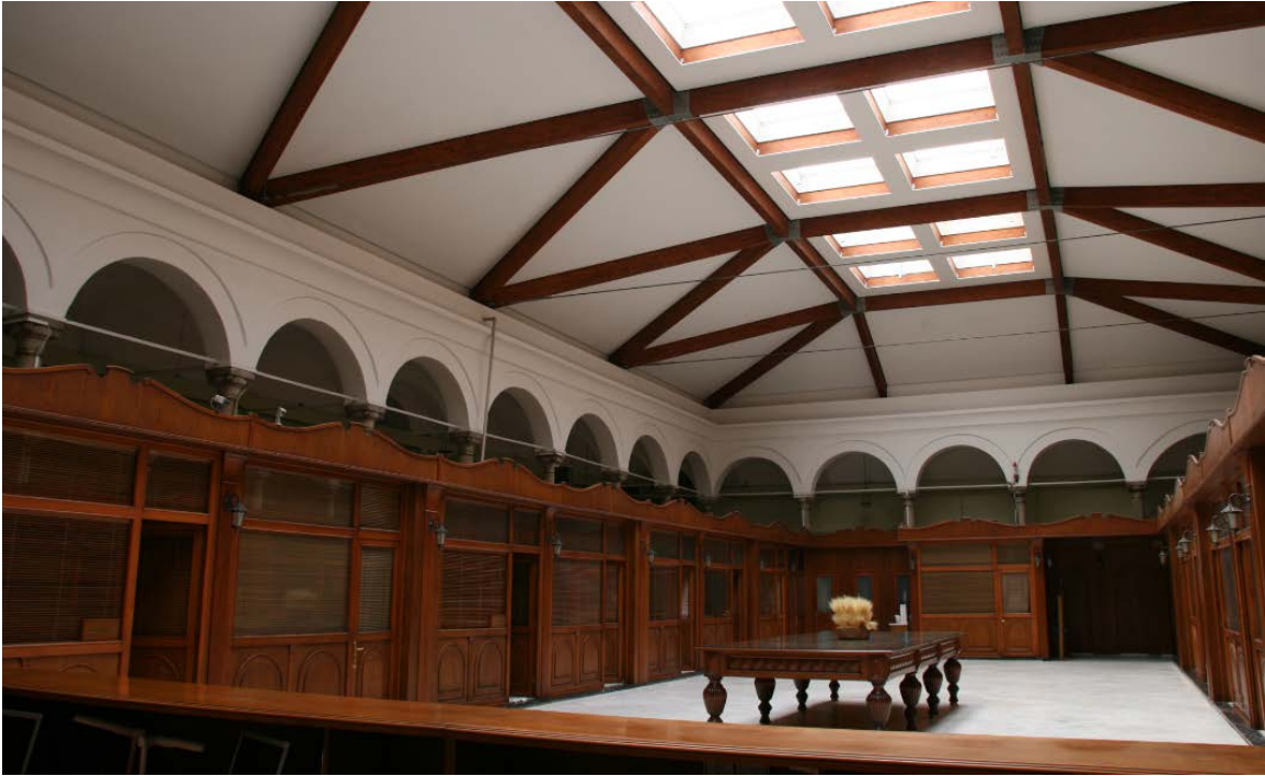
Figure 378. Hamidiye Complex, madrasa courtyard, now enclosed.
