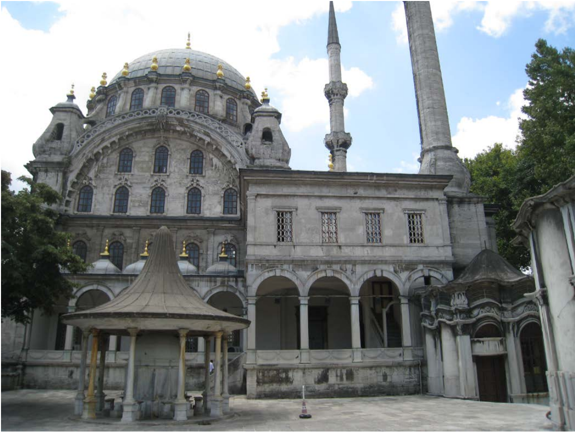
Figure 473. Nusretiye Mosque (architect: Krikor Balian), Tophane, Istanbul, 1823–26.
