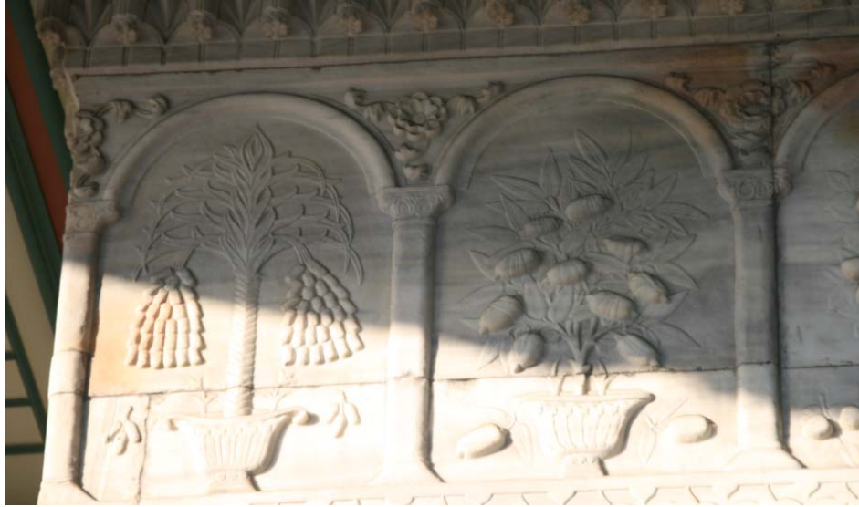
Figure 49. Fountain of Mahmud I, frieze along the top.
