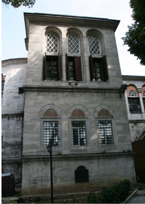
Figure 155. Nuruosmaniye Complex, sultan's pavilion, projecting room at the outer corner.
