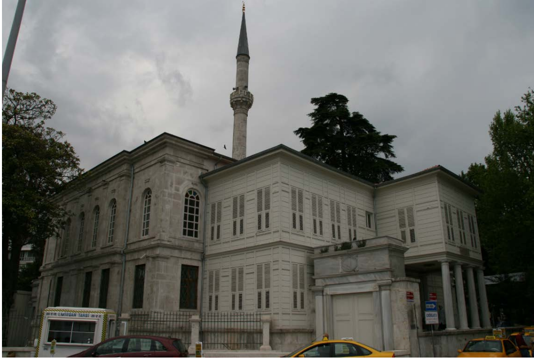
Figure 437. Emirgan Mosque, Istanbul, rebuilt 1838.
