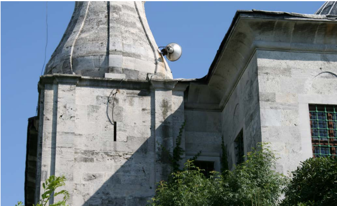
Figure 429. Beylerbeyi Mosque, view of the join between the minaret of 1810–11 and the existing sultan's pavilion.
