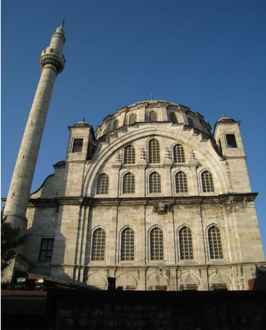
Figure 254. Ayazma Mosque, southwest facade.
