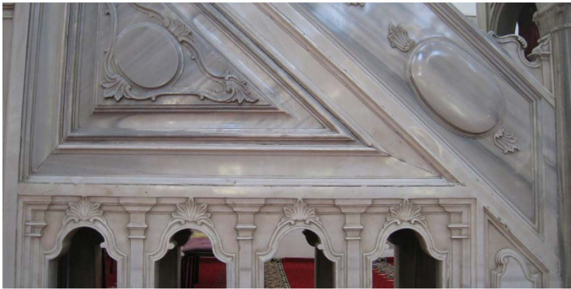
Figure 463. Selimiye Mosque, flank of the minbar.
