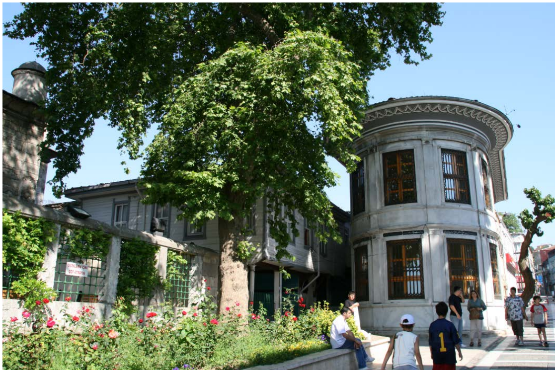
Figure 397. Beylerbeyi Complex, primary school (left, late-eighteenth century), and timekeeper's office (right, 1811–12).
