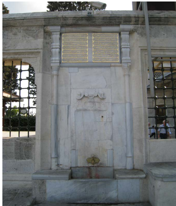
Figure 59. Inauthentic modern restoration of the fountain of Nişancı Ahmed Pasha, southwest wall of the Fatih Complex cemetery, Istanbul.
