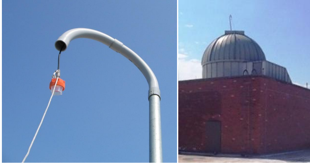
Figure 2-6. Sample inlet mounted above the observatory dome at the UMB site.
