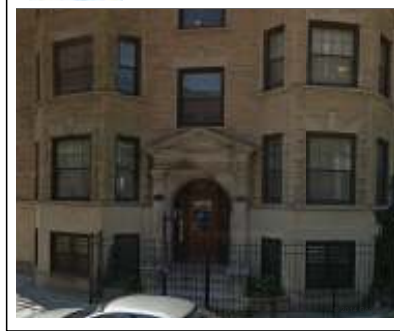
Fig. 10. Older large apt. building, well-kept 1019 W Foster Ave, Chicago, IL
