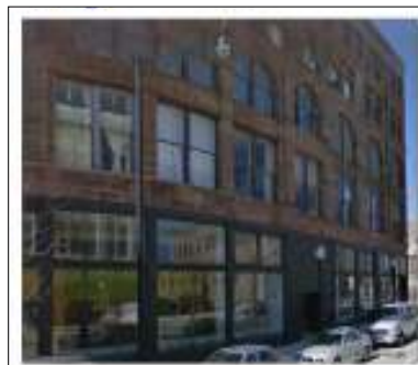
Fig. 15. Converted industrial use Address: 1962 South Halsted Street
