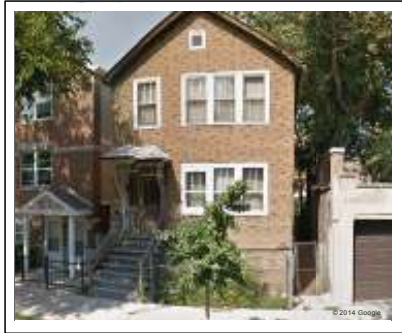
Fig. 1. Older residence and not well-kept in Chicago 1410 W Huron St, Chicago, IL
