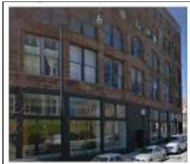
Fig. 3. Converted industrial use Address: 1962 South Halsted Street
