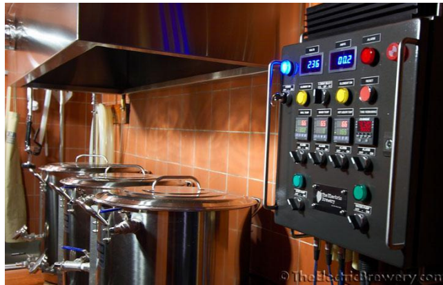
Figure 13 - Photo of The Electric Brewery (assembled)
