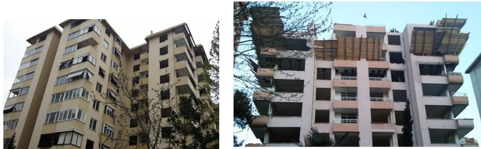
Figure 4.11: The multi-storey buildings demolished in the Kadıköy district.
