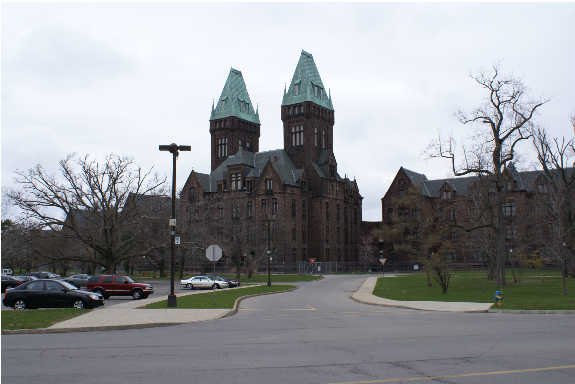
Figure 15. The Buffalo State Hospital: Long abandoned, the building is currently undergoing stabilization treatment (Photo by author).
