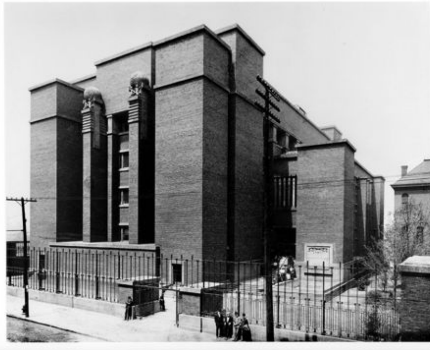
Figure 3. The Larkin Administrative Building. Image from: The Hydraulics Press , Url: http://www.hydraulicspress.org/the_hydraulics/2009/05/newsweek-puts-spotlight-on-larkin-administration-building.html .
