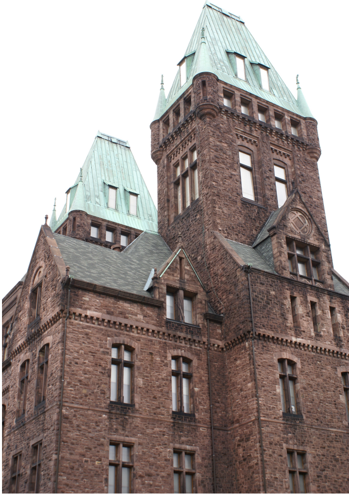
Figure 16. Richardson's Towers: notice the fenestration banding, something Wright also designed into his several Buffalo houses- could he have been emulating Richardson? On other parts of the building, Richardson cascades the fenestration where it parallels interior stairways. This nod to the functional elements of the building would have impressed Sullivan (Photo by Author).
