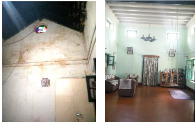
Figure 29. House 2(left) and House 1(right) with clerestory windows emitting light into the high ceiling area.
