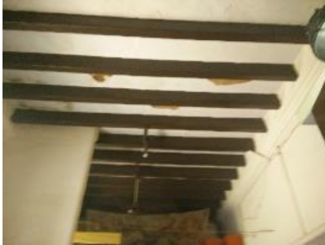
Figure 8. Photo of Madras terrace roof.
