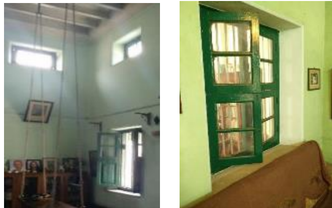
Figure 30. House 1 with deep set windows with wooden frames and grills and high ceiling height.
