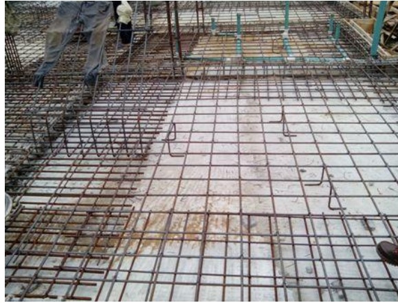
Figure 10. Construction of an RCC slab.
