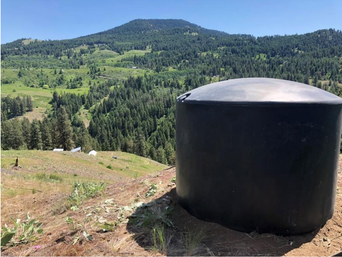
Figure 4. Uphill 1500-gallon water tank with bottom tank downhill in picture to the right of buildings (photo by author, 2018).
