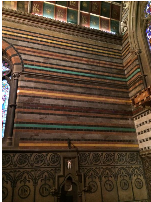
Figure 3.9 North wall detail of chancel stripe pattern.
