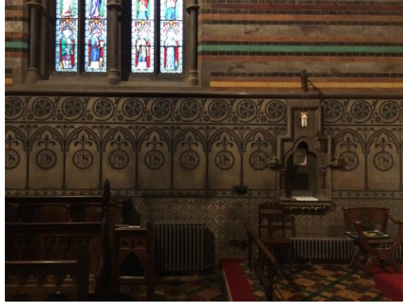
Figure 3.11 North wall of the chancel of All Saints Boyne Hill, featuring an aumbry (right) with similar stenciled patterns on each side.
