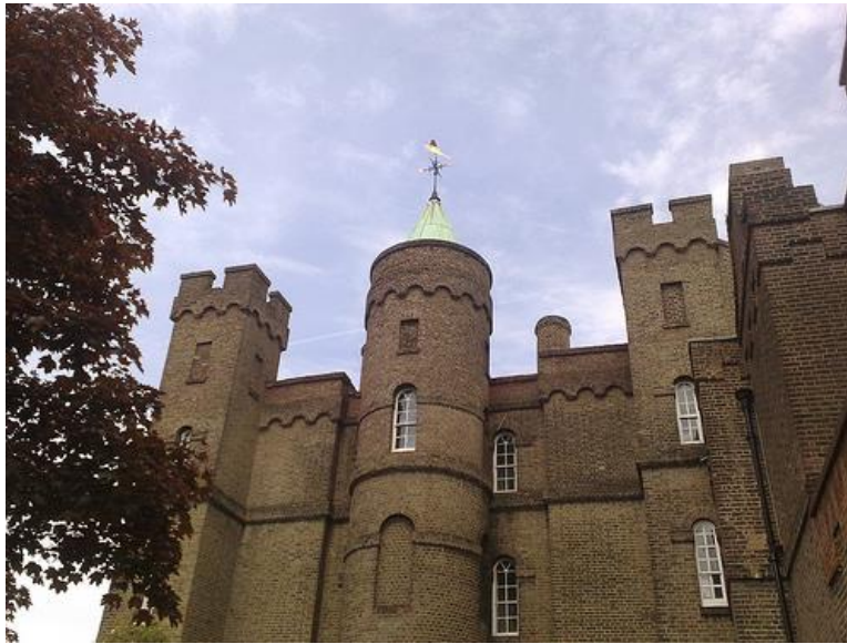
Figure 1.18 Vanbrugh's own castle at Greenwich (1719), features shallow decorative machicolations and overscaled crenellations at the corner towers. If it was still fairly outside mainstream taste to treat castles as serious architecture in the late eighteenth century, it was doubly idiosyncratic to do so in the seventeenth. Yet Vanbrugh did champion the castle type, designing several projects in this idiom for himself and one for an adventurous client, and arguing unsuccessfully to preserve the ruins of a genuine medieval structure on the grounds of the Duke of Marlborough. Vanbrugh shared Clerk of Eldin's sentiment that castles were architectural-scale indices of the passage of time, and his castles feature round and Diocletian windows and crosslet loops, just as Adam's do. He also seems to have seen his castles as a hybrid between the landscape-like irregularity of ancient keeps and the symmetry and proportion required of modern architecture since the classical era. 84
