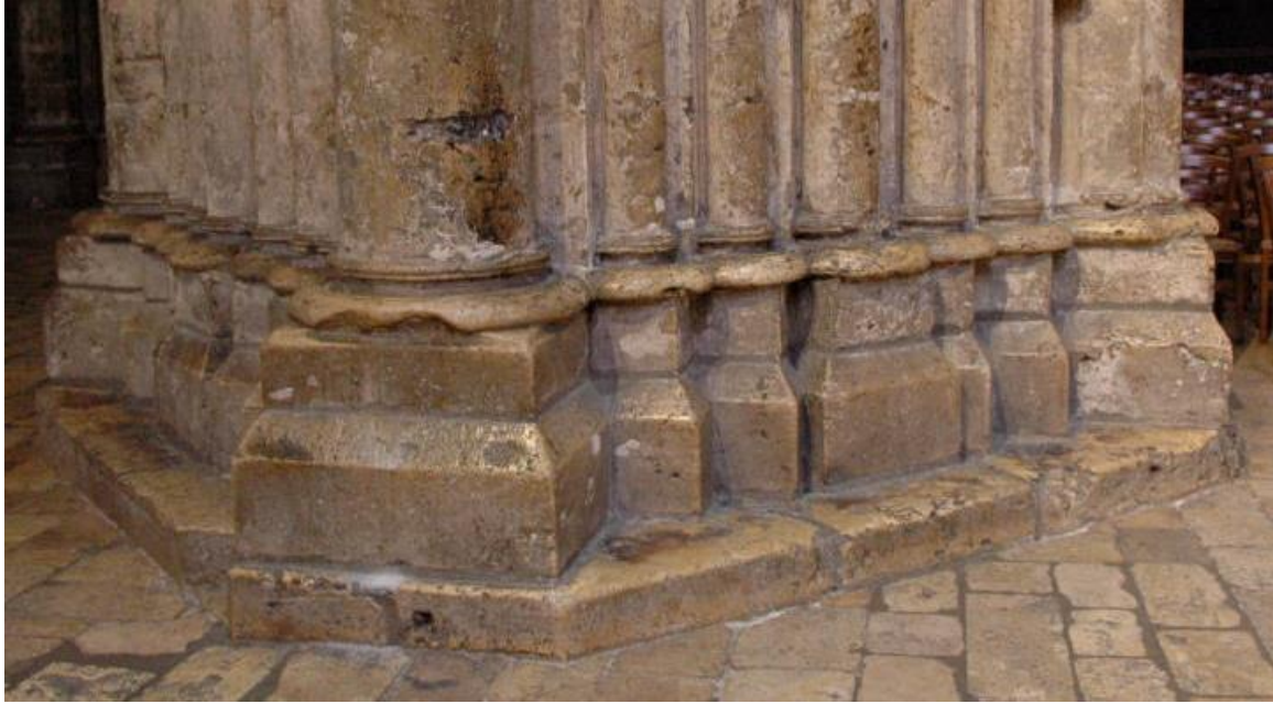
Figure 4.7 A “crystalline” column base at Abbeville Cathedral.
