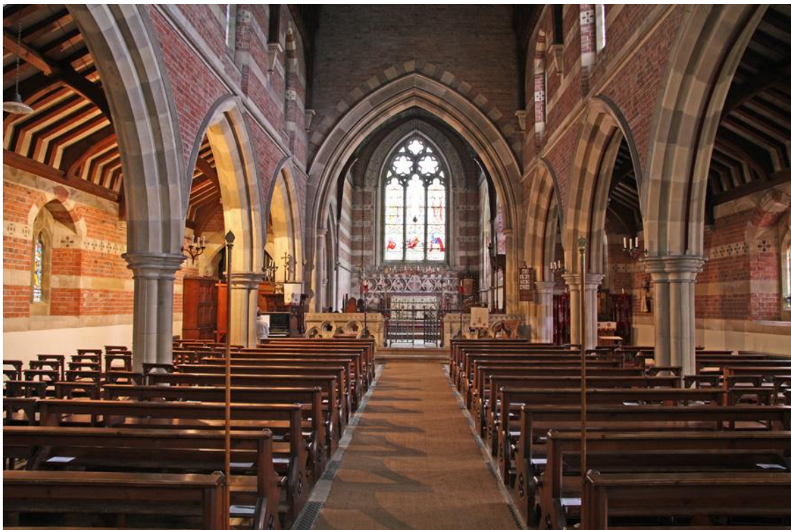
Figure 3.20 William Butterfield, interior view of the parish church at Baldersby St. James, North Yorkshire. In Butterfield's design, the sill band that runs along each side of the nave terminates into the chancel arch – a typical design solution for the time. At Boyne Hill, such a resolution is actively avoided. See Figure 3.13.
