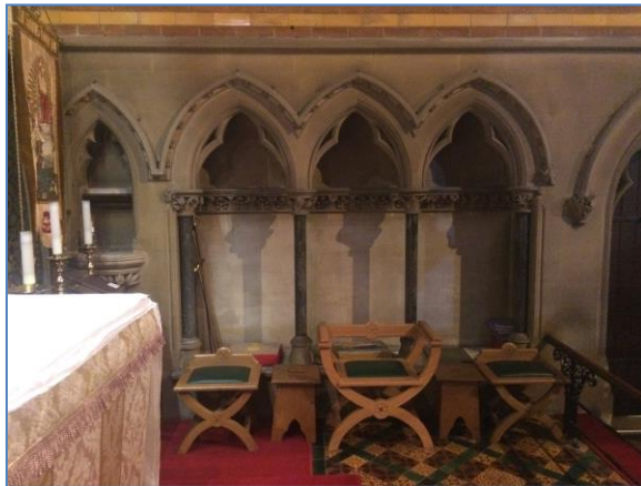
Figure 3.10 G. E. Street, south wall of the chancel of All Saints Boyne Hill, stone group of piscina and credence shelf (left), sedilia (center), and vestry door (only partially visible, at right).
