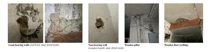
Figure 4-74 Brick-wood structure of building No. 29 and building No. 30
