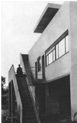
Figures 4.54, 4.55, 4.56 and 4.57. Housing Settlement in Pessac, Le Corbusier, 1925-1926.
