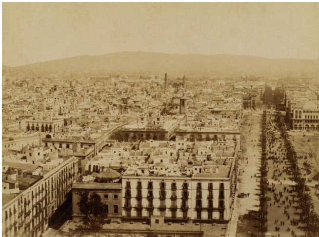
Figure 2.23. Aerial view of Ciutat Vella, Barcelona, 1880s . Photo by Antoni Esplugas.
