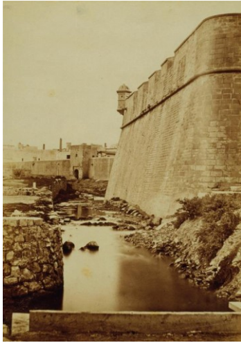
Figure 2.20. The old wall, Desconegut, Barcelona, 1860s.
