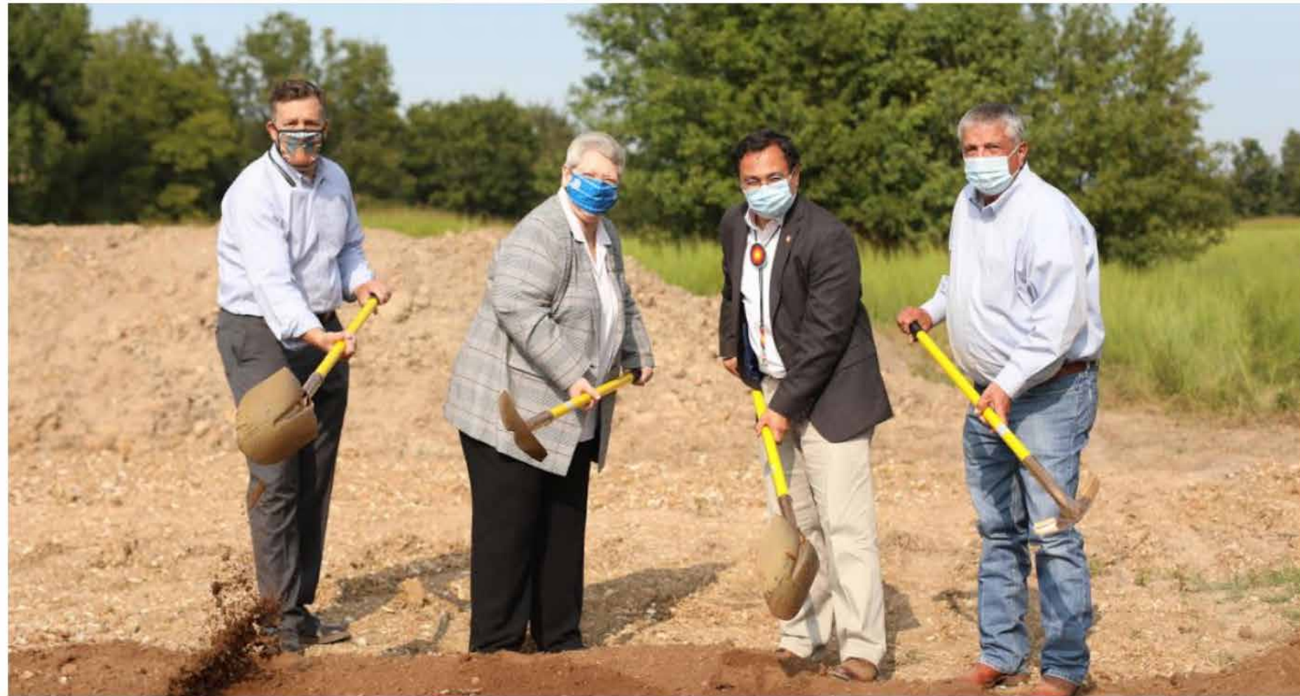
Cherokee Nation Chief of Staff Todd Enlow, Secretary of State Tina Glory Jordan, Principal Chief Chuck Hoskin Jr. and Tribal Councilor Rex Jordan break ground in Hulbert on Sept. 8 at the future site of a PPE manufacturing facility.
