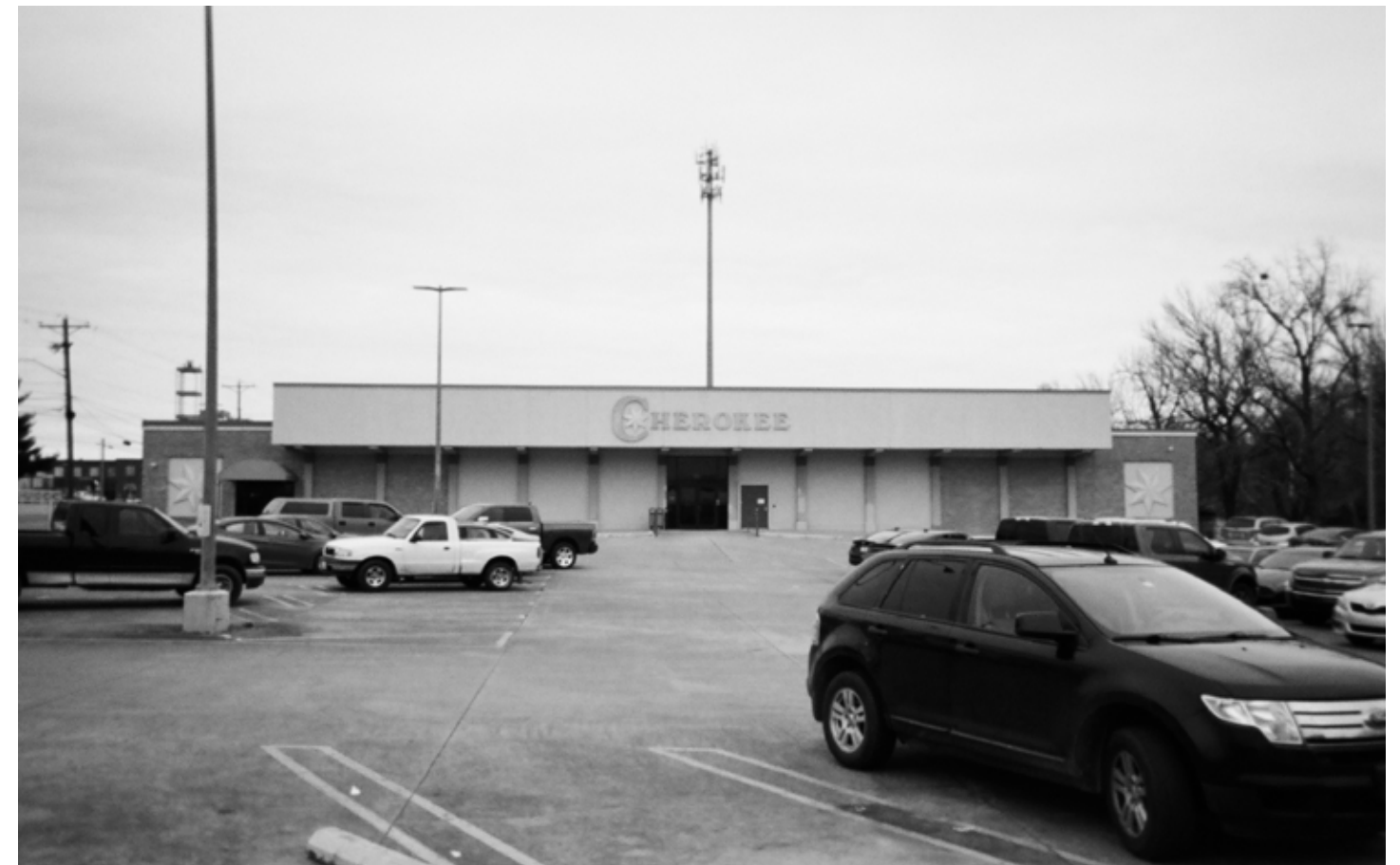
Image 29: Cherokee Offices in former Grocery Store, January 2021
