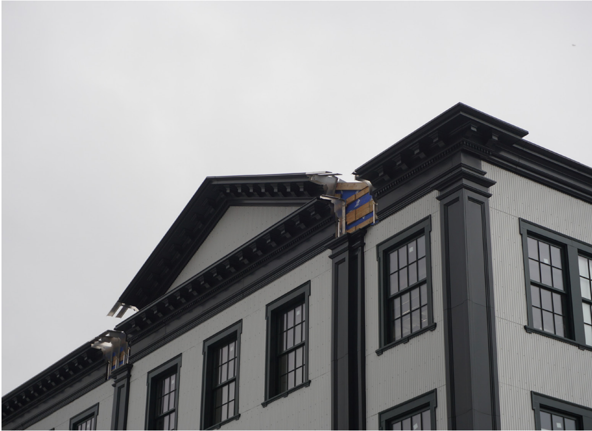
Tin Building in construction Jan. 15, 2021.
