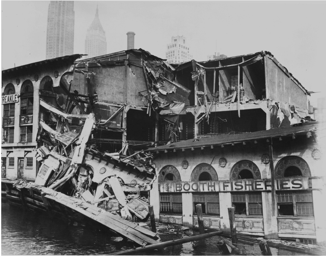
Fulton Fish Market collapse, 1936.
