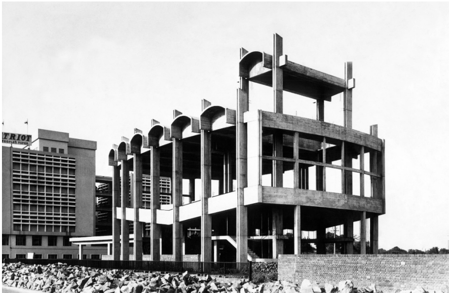
Figure 27: Concrete frame of Gandhi Memorial Hall; photograph by Madan Mahatta; [from the Mahatta archives]
