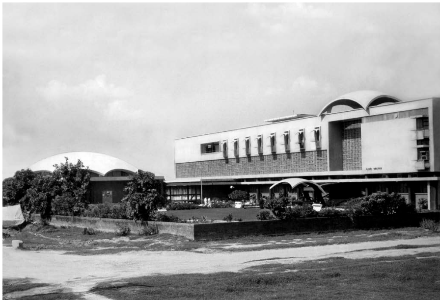
Figure 20: Azad Bhavan from the main road; [from the Kanvinde, Rai & Chowdhury archive]
