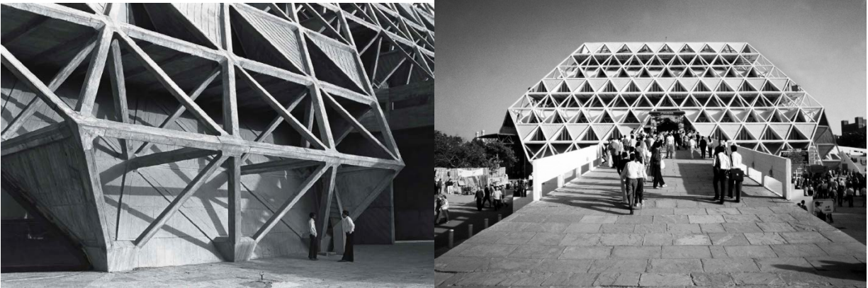
Figure 52: Springing point of the tetrahedron structure; elevation of Hall of Nations
