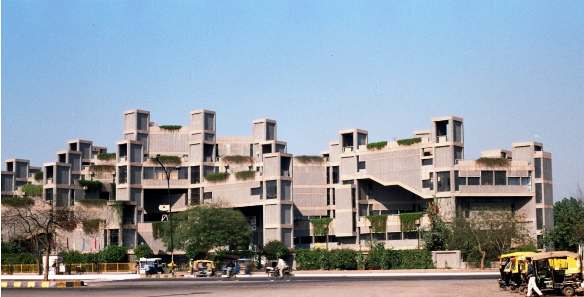
Figure 55: The National Science Centre as seen from Bhairon marg; [from the Kanvinde, Rai & Chowdhury archive]
