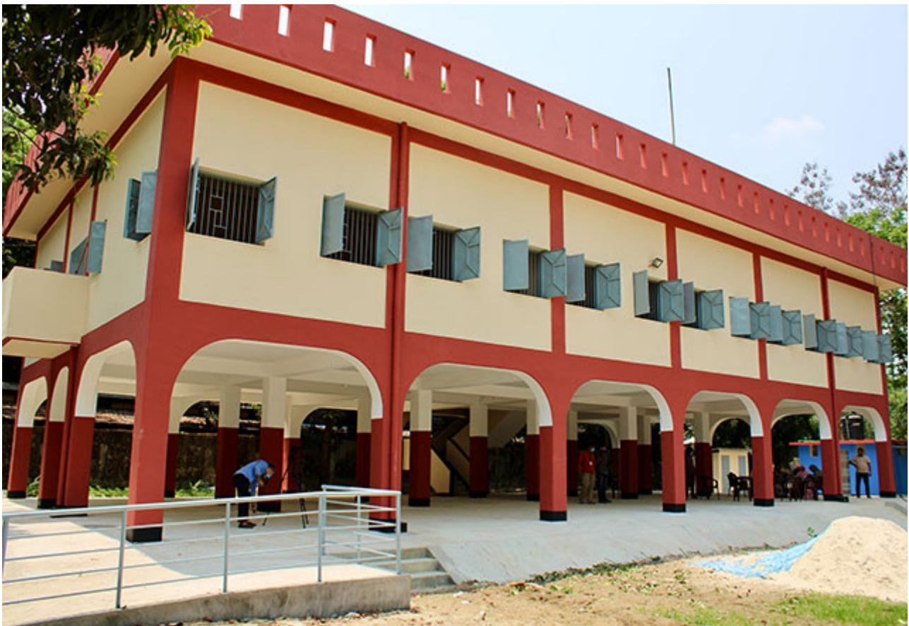
Figure 3. Cyclone shelter in southeastern Bangladesh. Note the elevated shelter structure and the use of columns that allow floodwaters to pass without damaging the structure.
