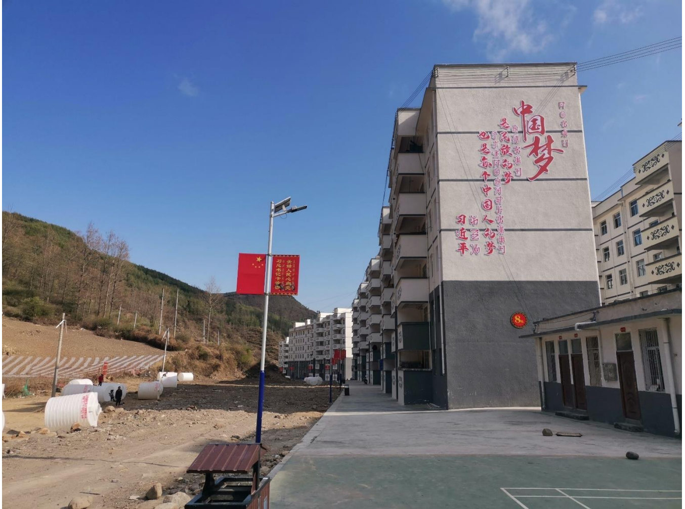
Figure 3.2. Newly constructed apartment buildings in Hongxi town. Many people from nearby villages have been relocated to here. The characters on the wall say “The Chinese dream is [our] people’s dream, and also every Chinese person’s dream” by current CCP president Xi Jinping.
