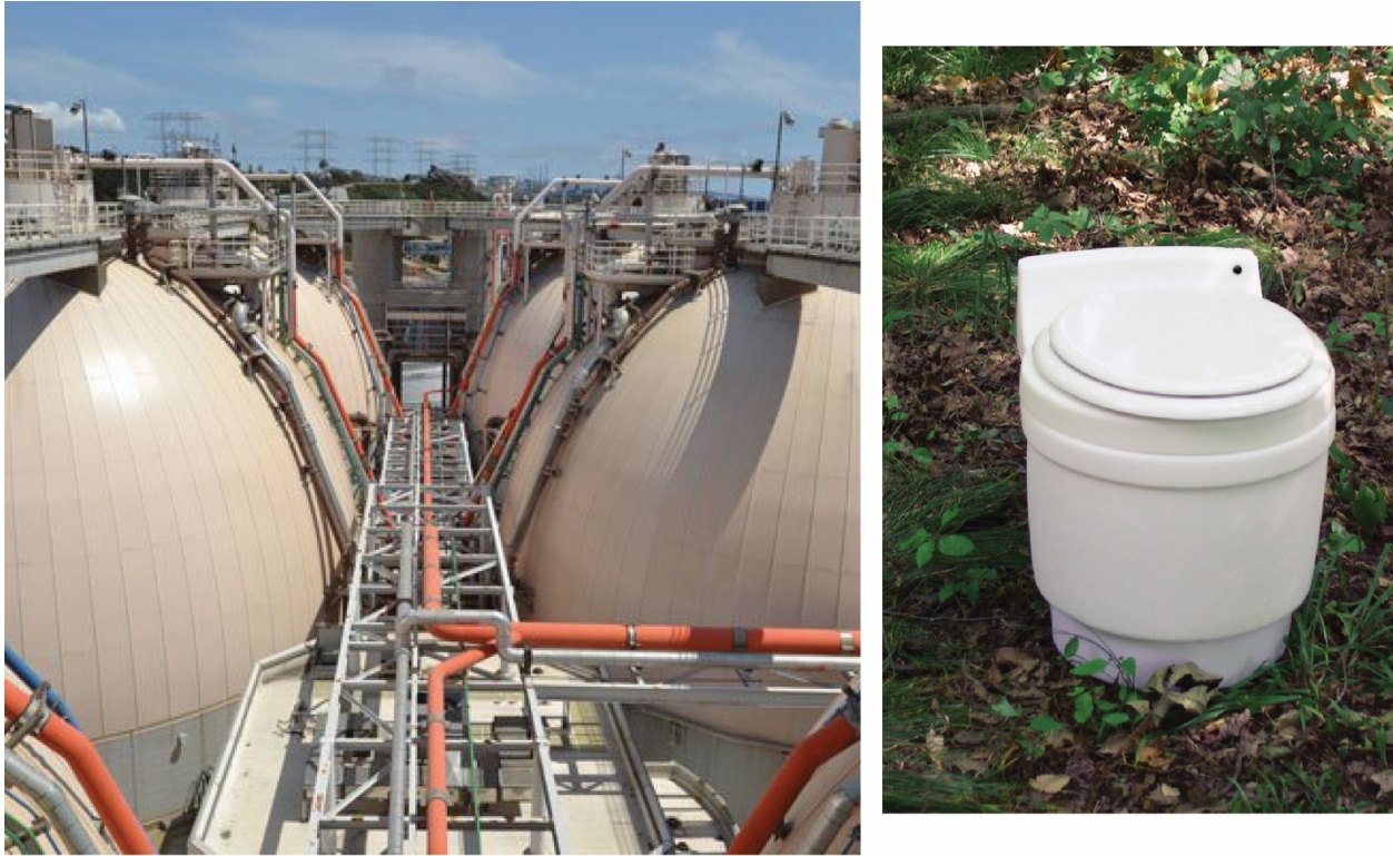
Fig. 6. 6 The Hyperion sewage treatment plant in Los Angeles (left), a composting, waterless toilet (right).
