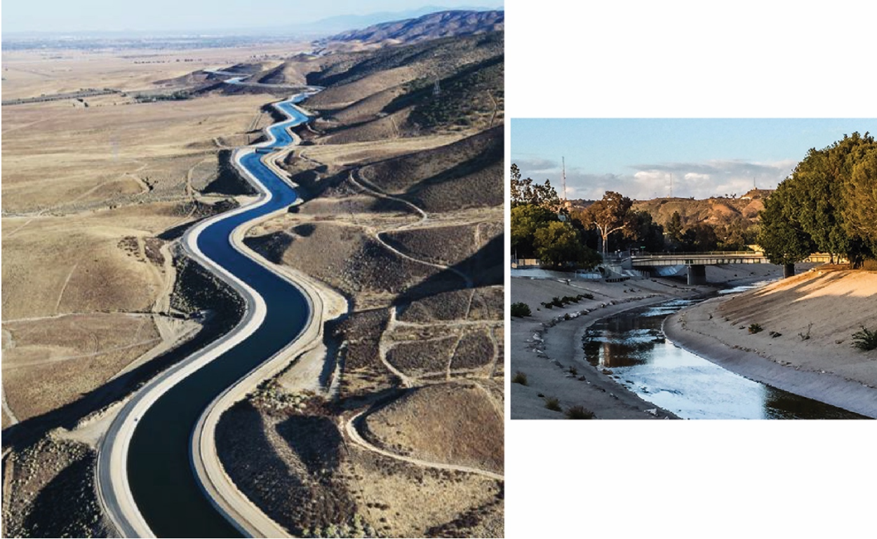
Fig. 6. 5 Los Angeles Aqueduct (left), the Ballona Creek flood-protection channel which drains water from the L.A. basin to the ocean (right).
