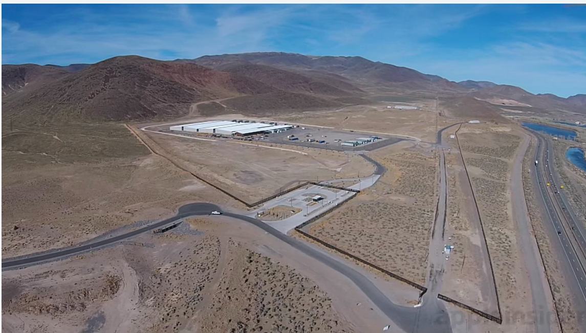
Figure 3.2: Apple's Reno Datacenter in 2015.
