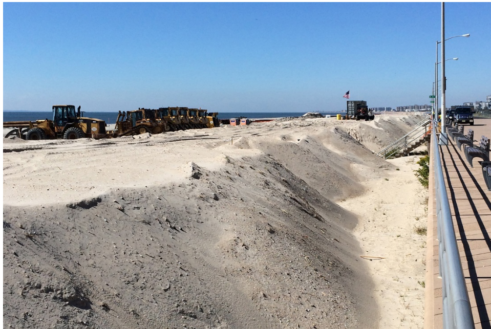
Figure 45. Sand dune construction to prepare for storm surge.
