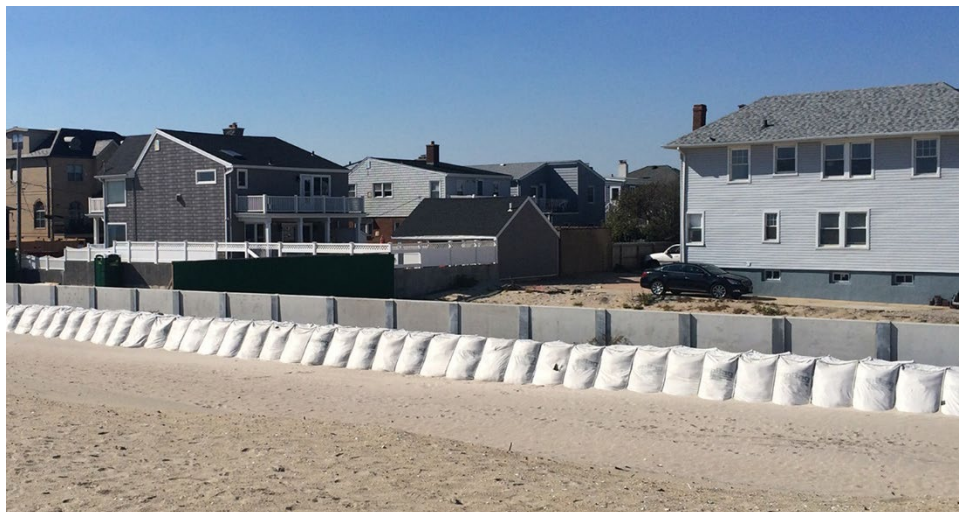
Figure 43. Storm surge barrier construction.
