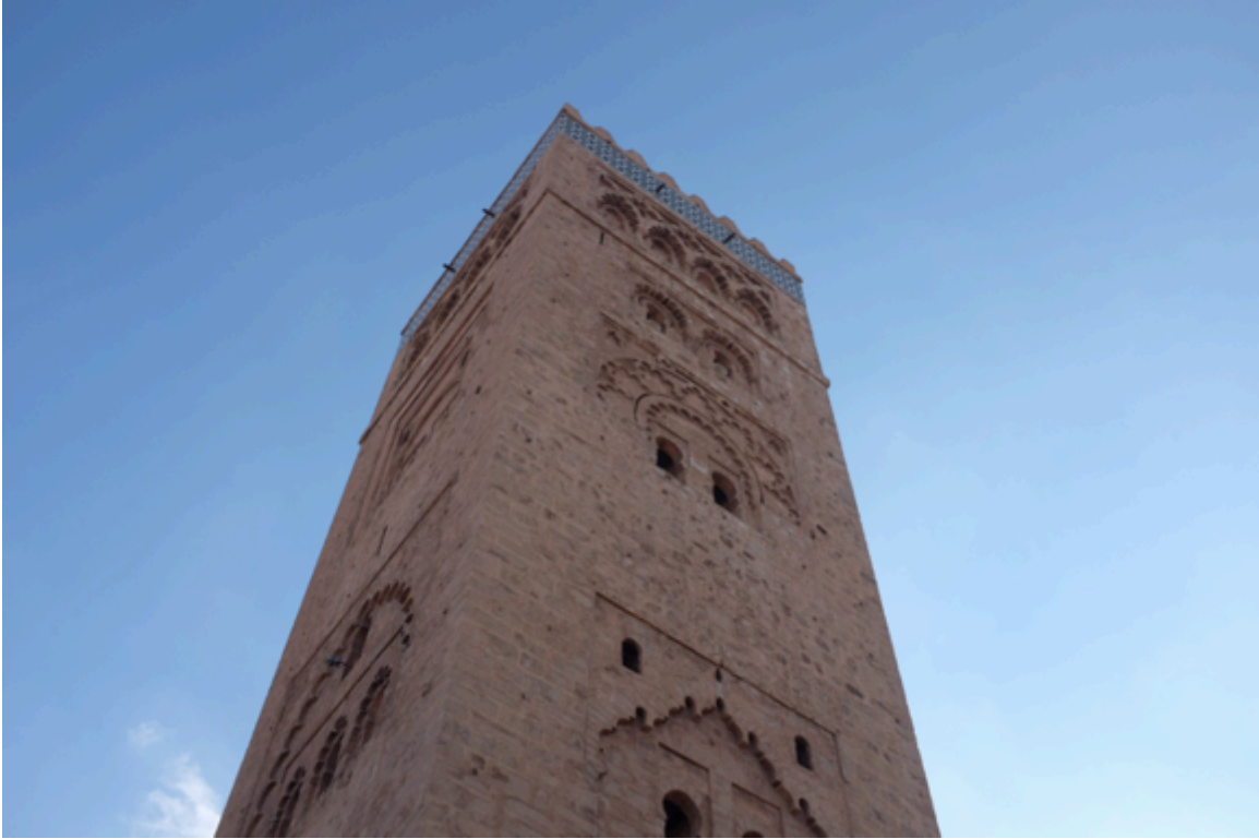
Fig. 2.29: Staggered alfiz registers on the northeast and southeast faces. Photos author's own.
