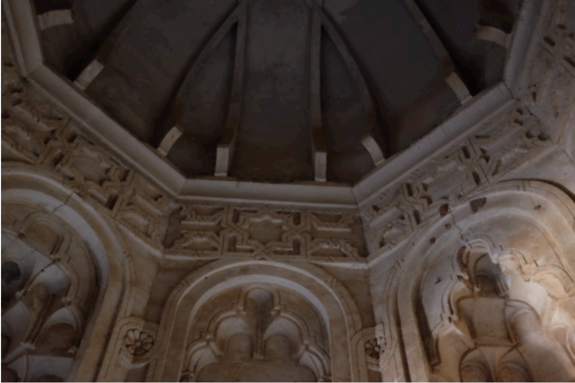
Fig. 2.31: Uppermost chamber within the minaret. Photo author's own.
