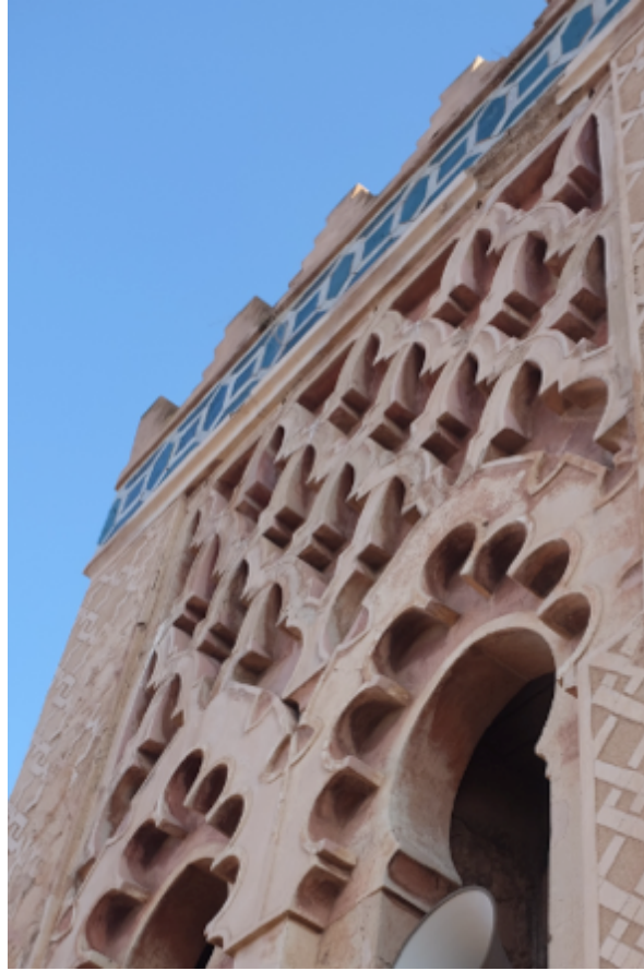
Fig. 2.33: Residual red paint within the interstitial spaces of the arcature. Photo author's own.
