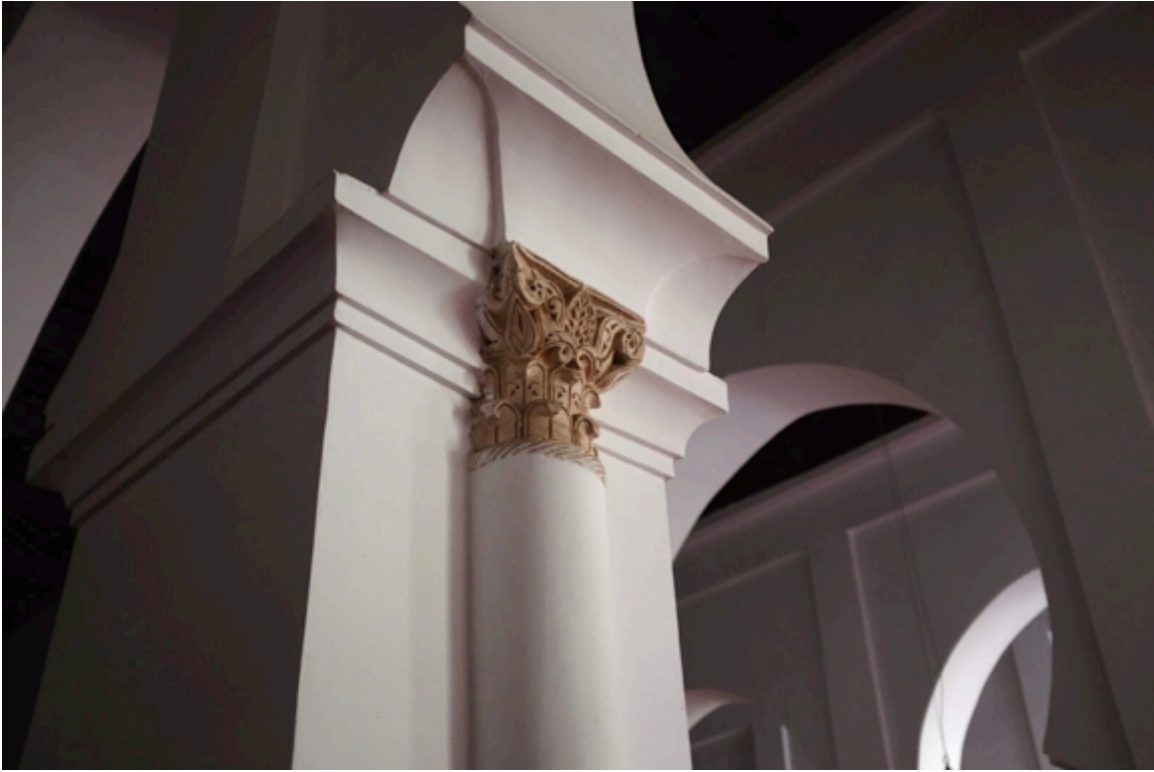
Fig. 2.7: Engaged column with stucco capital in the second Kutubiyya prayer hall. Photo author's own.
