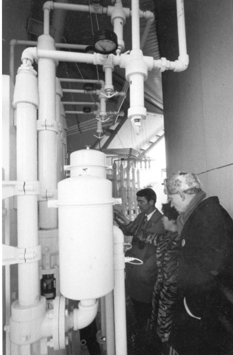
Figure 4.31. Pump installation for fog system, Pepsi Pavilion, 1970; Fujiko Nakaya and Billy Klüver. Reprinted from E.A.T., Pavilion (New York: E.P. Dutton, 1972).
