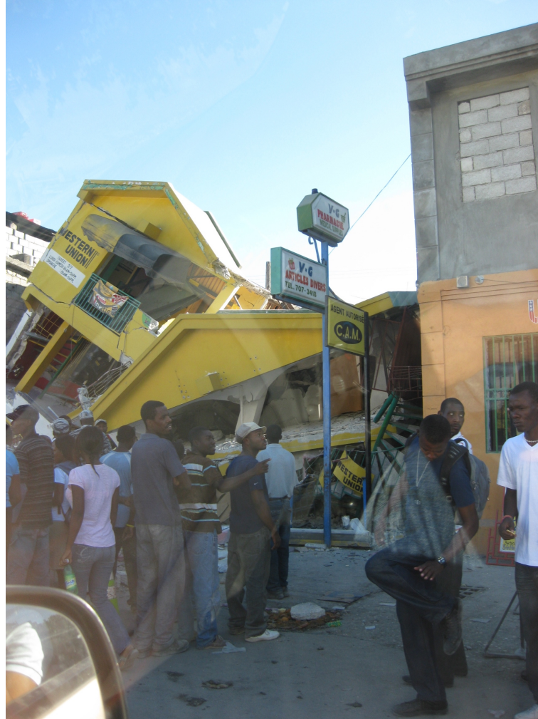
Figure 2. Photo taken by Lucien Rousseau of crumbled buildings after the 2010 earthquake in Haiti.
