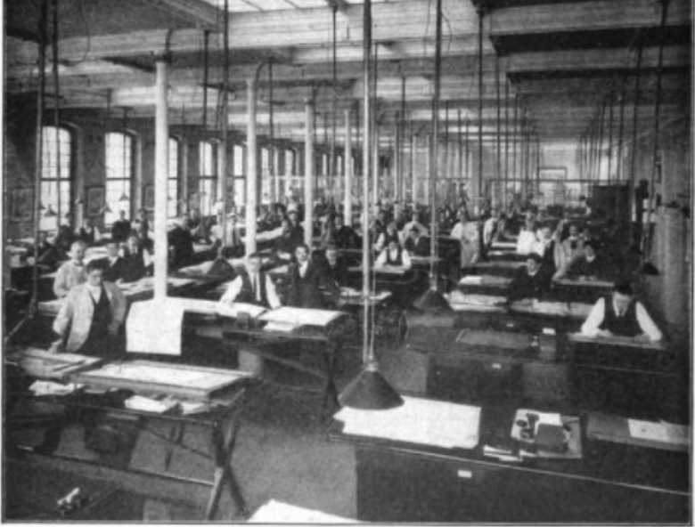
THE DRAFTING ROOM OF THE BROWN & SHARPE CO., PROVIDENCE, R. I.
