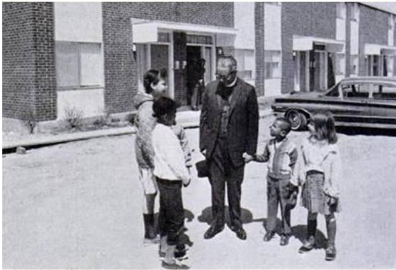
Charlame Apartments in Boston is a 92-unit development completed this spring under sponsorship of Charles Street A.M.E. Church. The two- and three-floor townhouses are of brick veneer construction, have two-, three- and four-bedroom units that rent for $88, $98 and $108 monthly. The church's pastor, Rev. Walter C. Davis, talks with resident children.
