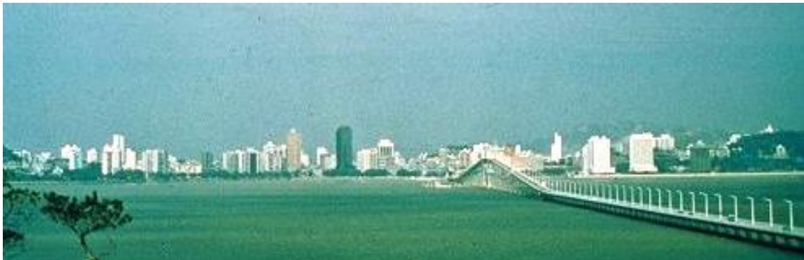
Figure 2.18: Landfill Zone of Porto Exterior seen from Taipa. Hotel Presidente and Hotel Lisboa located on the right side of the Governador Nobre de Carvalho Bridge, 1976 (Source: Vanessa Seed and Manuel Noronha)
