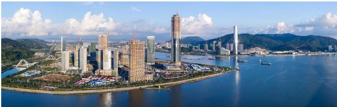
Figure 4.14: The aerial view looking towards northwest of the Cross-Gate CBD in construction. 2018. (Source: Kevin Zhen)
