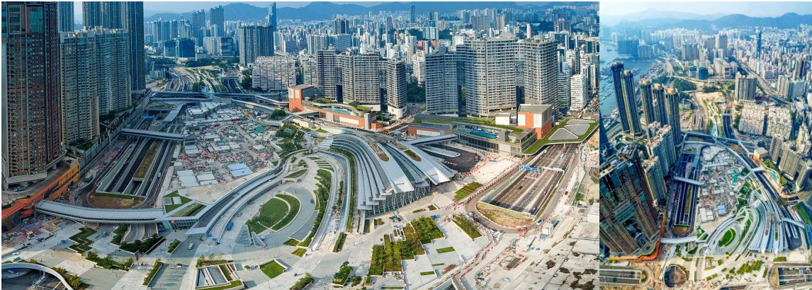
Figure 5.3: Aerial view of the West Kowloon Station Terminus and the Union City development on its left. 2018 (Source:Asean)
