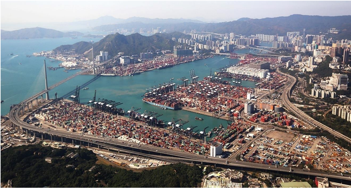
Figure 5.22: The aerial view of Kwai Tsing Container Terminals. (Source: Survey and Mapping Office, Lands Department. The Government of Hong Kong Special Administrative Region.)
