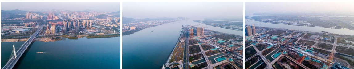
Figure 4.3: The aerial view of Bay Pioneering Zone in construction, with the Lingshan Island as the future urban center. 2016. (Source: Sohu Images)
