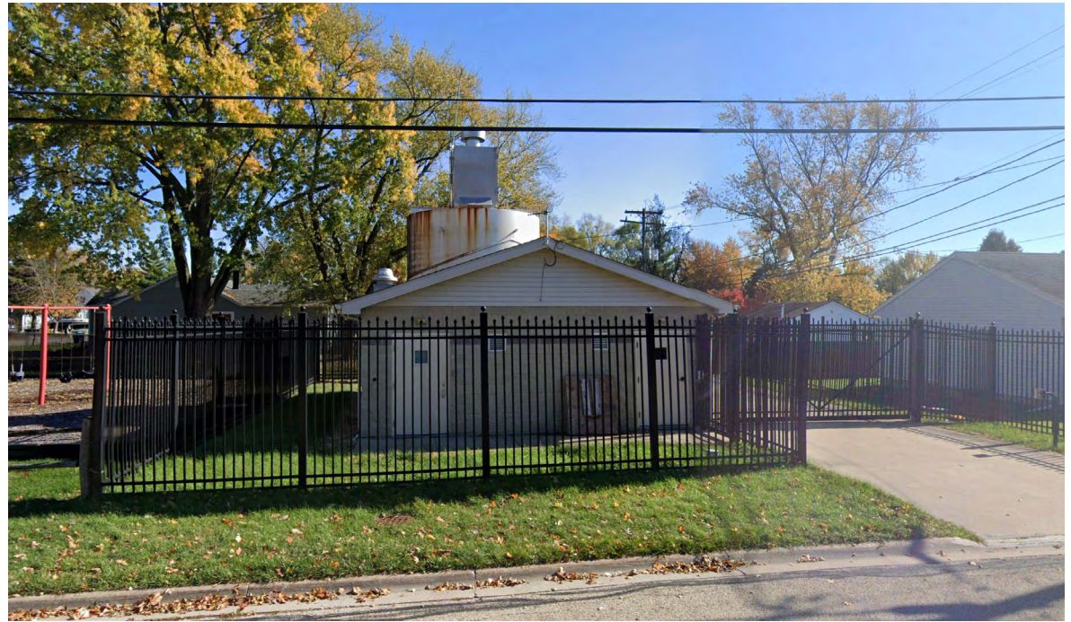
Existing condition of the small site
