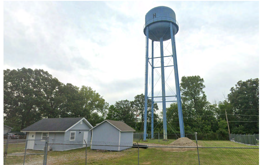
Existing condition of the medium site
