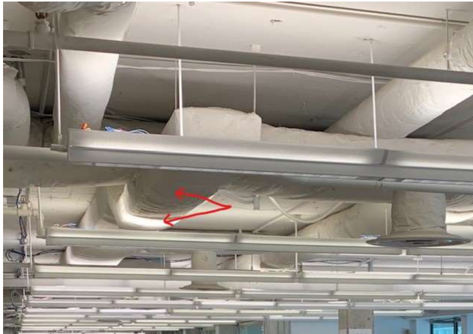
Figure 35. Example of ceiling luminance ratio exceeding requirements of Feature L06. Red arrows point to two sections of ceiling where the ratio is greater than ten times greater or lesser luminance June, 2019.
