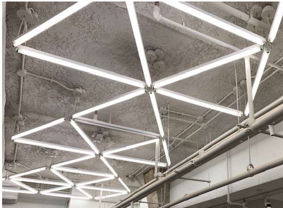
Figure 30. Photograph of the fixtures that would have prevented the MOS from achieving Part two of Feature L04 due to a high UGR.
