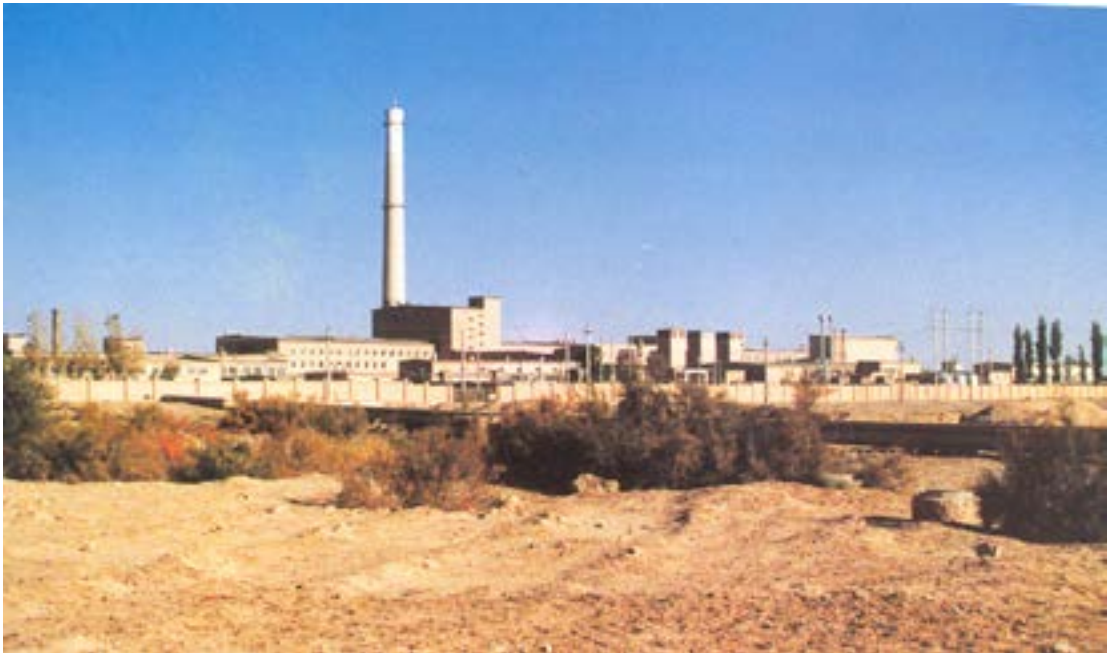
Figure 2.4: The Pilot Civilian Reprocessing Plant at the Jiuquan Nuclear Complex
