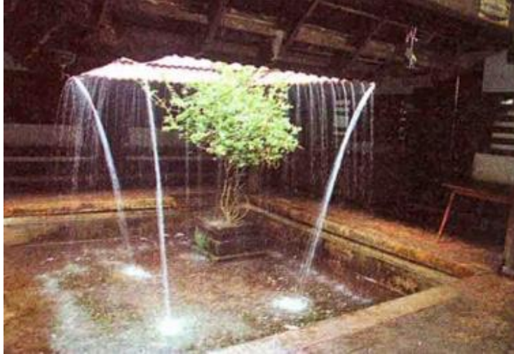
Figure 15. Courtyard used for rainwater harvesting (Lakshamanan, n.d).
